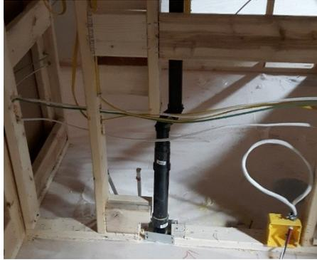
Figure 1-2: Cutting and reinforcement of wall studs
