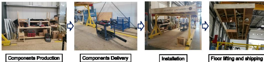
(b). Drainage system prefabrication on framed floor panels
