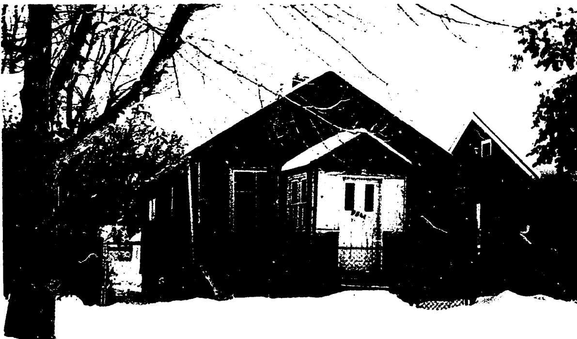
Photograph 1. Evidence of Disinvestment and Neglect in Rossdale's Older Housing Stock
