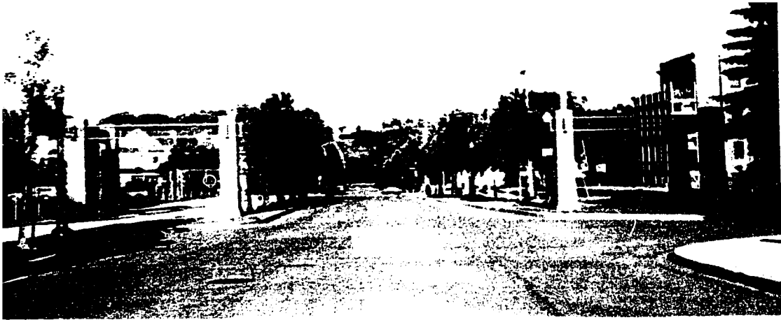
Photograph 2. Rossdale's Main Entrance: Example of streetscape and infrastructure improvements including new curbs, sidewalks, brick and iron gages, and park benches
