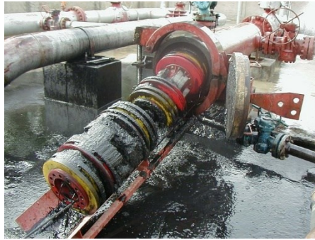
Figure 2.5: Pipeline pigging system
