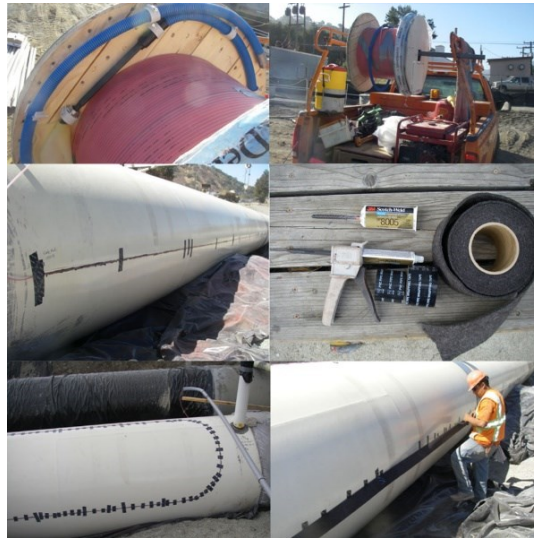
Figure 2.7: Installation of a fiber optic leak-detection cable
