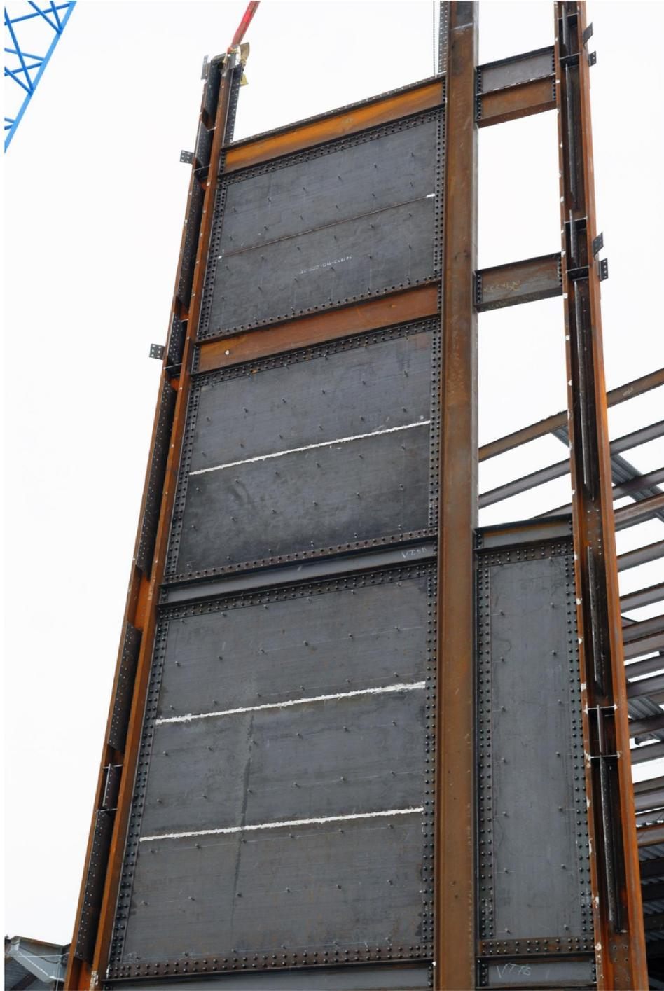
*Figure 1.5 - Edmonton International Airport Control Tower Steel Plate Shear Wall
