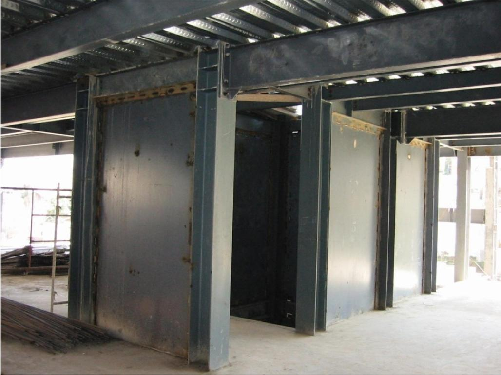
*Figure 1.7 – 22-Storey Condominium Steel Plate Shear Wall in Mexico (Courtesy of Martinez-Romero, 2003)*
