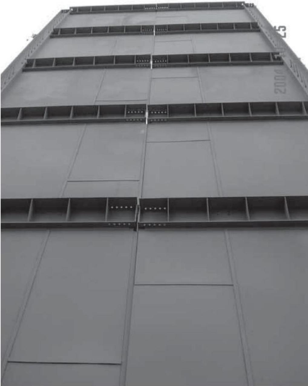
*Figure 1.3 - SPSW Mid Span Splice, ING Building (Courtesy of Group Teknika)*
