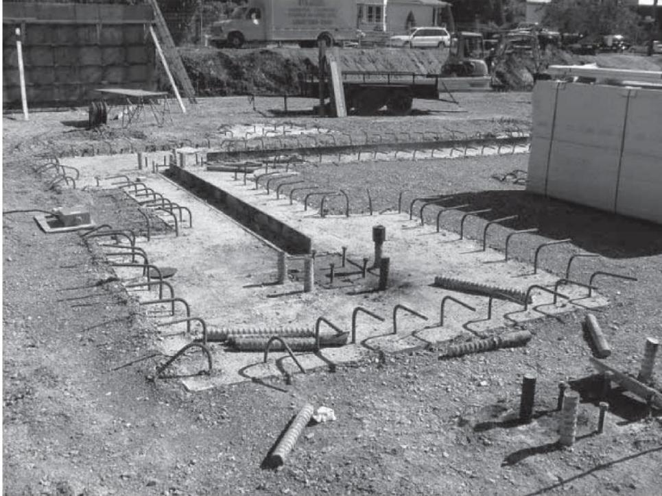
*Figure 1.4 - Steel Plate Shear Wall Base Anchorage, ING Building (Courtesy of Group Teknika)*
