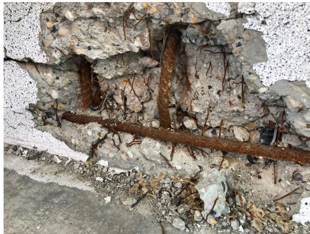
Figure 2-2: Concrete column with corrosion resulting in exposure of steel reinforcement
