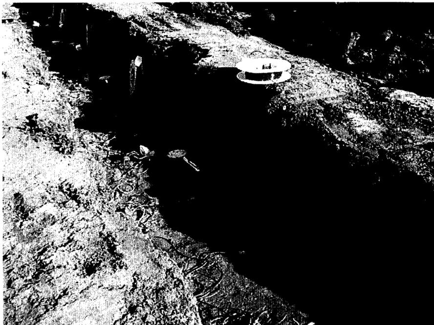
Figure 155: Picture of total pressure cell field installation
