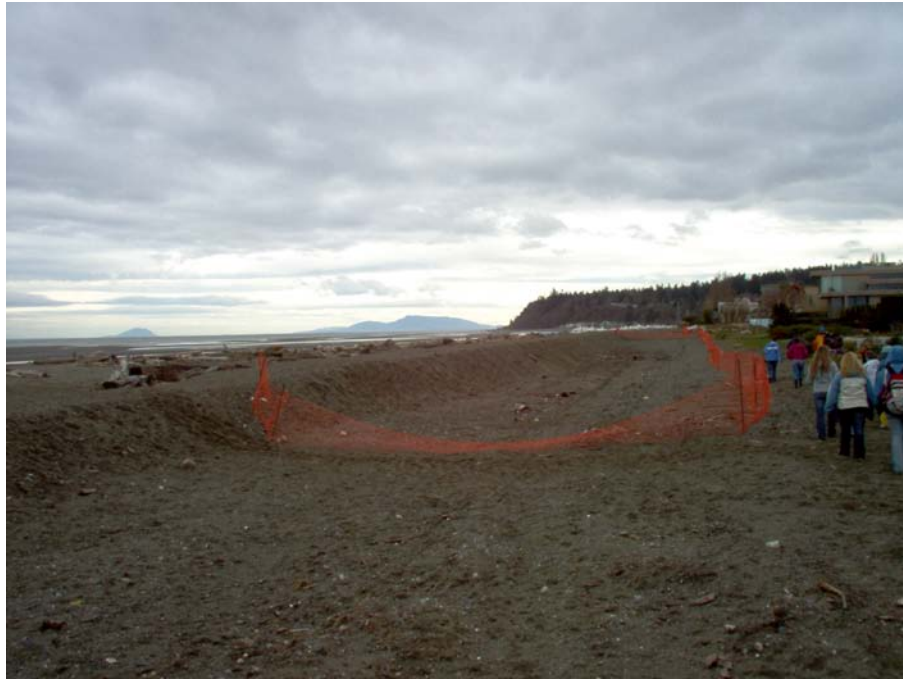
Figure 12 Photo of the Berm (and trench) that protect homes in Boundary Bay Village
