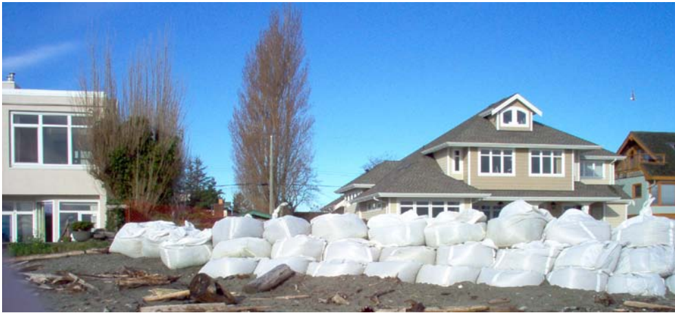
Figure 14 Photo of large-scale sandbags that protect homes south of the berm in Boundary Bay Village
