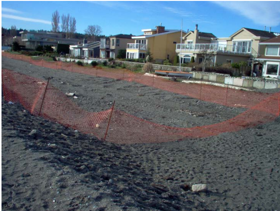
Figure 13 Photo from the top of the berm facing homes in Boundary Bay Village
