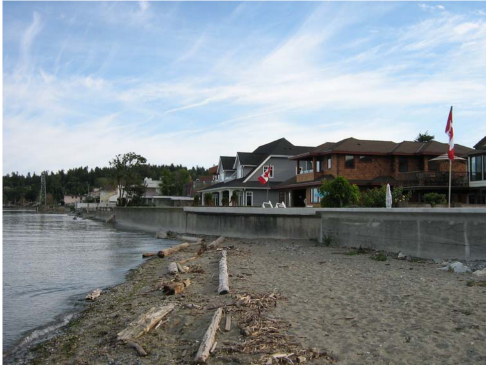
Figure 7 Photo of seawalls built along the southern coastline of Boundary Bay Village
