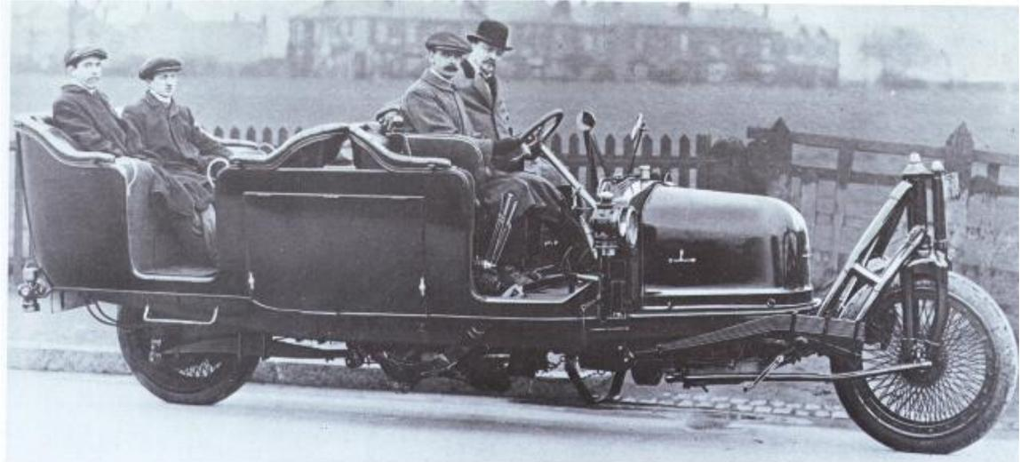
seemed convincing.<sup>58</sup> The vehicle weighted 2.75 tons on two wheels, which was not promising for the muddy Eastern Front. The vehicle was also said to suffer from a very large turning radius, which was also not favorable as a proposed military vehicle.<sup>59</sup> After the First World War broke out in the same year, Shilovsky returned to Russia and the project was never pursued any further.<sup>60</sup>
