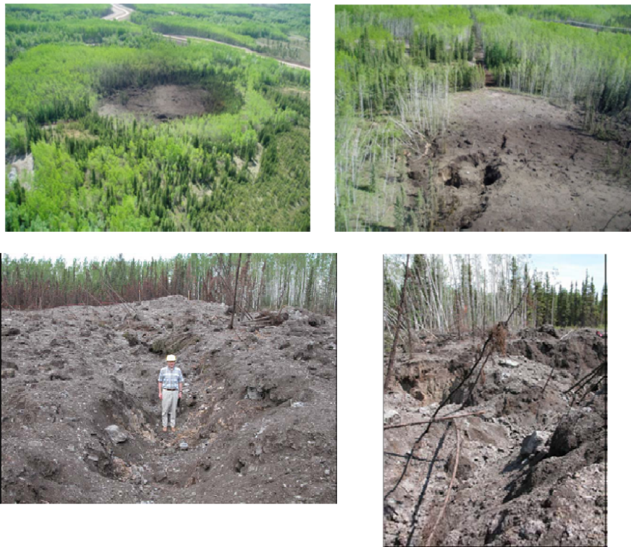
Figure 3-15 Steam release incident from Total’s report
