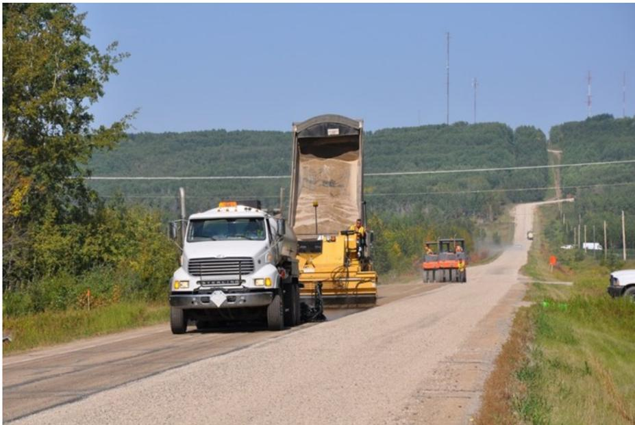
**Figure 1.2** Example of a pavement preservation application called “chip sealing.” The white truck in front first sprays a layer of bitumen emulsion (approx. 2 mm in thickness) onto the distressed pavement; it is closely followed by a second truck which deposits aggregates (small rocks) onto the sprayed emulsion layer. Trailing behind at a greater distance is a roller truck for compacting the composite structure.
