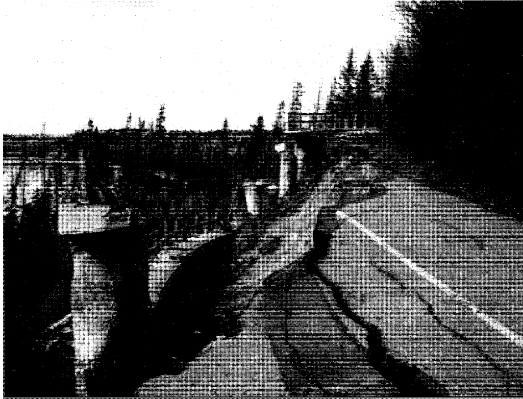
Figure 7-22 A photograph of the damaged pile wall at the Keillor Road Landslide (May 2004)
