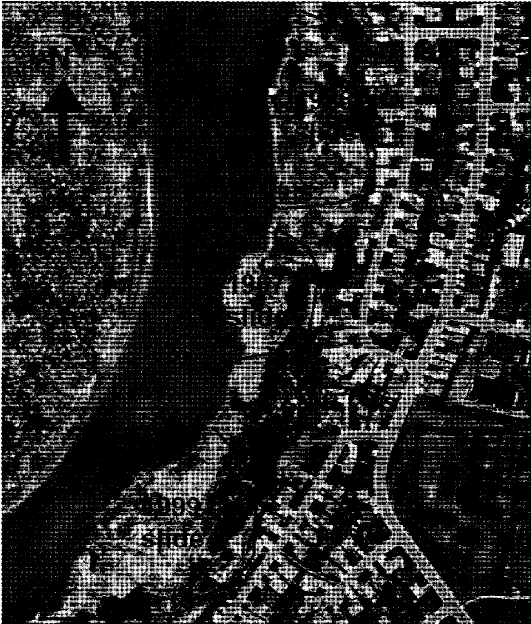
Figure 8-3 Landslides along Whitemud Road (May 2002, the City of Edmonton, Line 17E, Scale 1: 5000)
