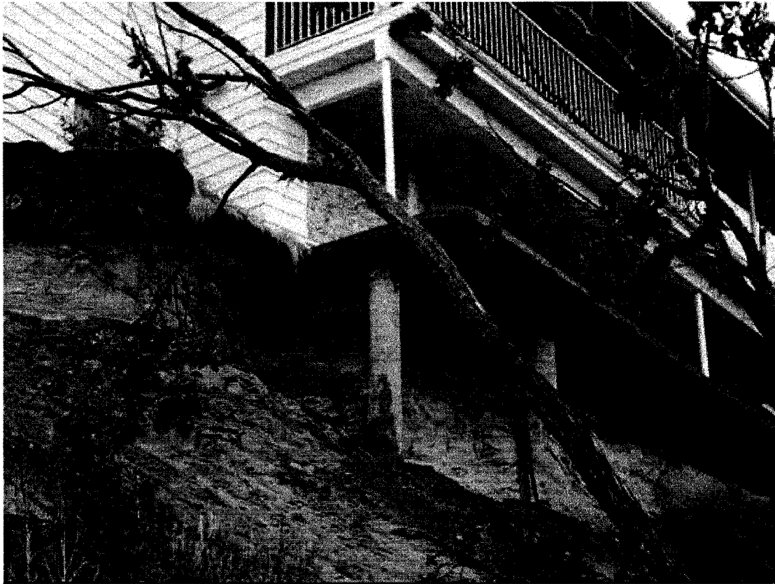
Figure 8-2 Photograph of exposed piles on lot 5 (November 1999)
