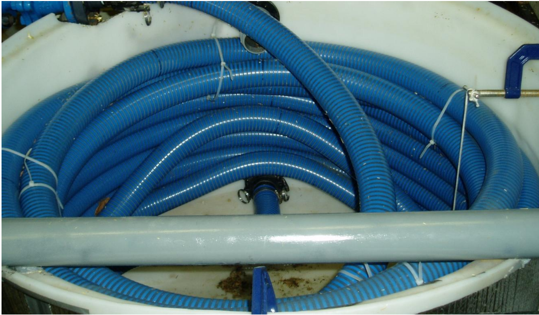
Figure 24: Coils of long radius hose in line with pipeline
