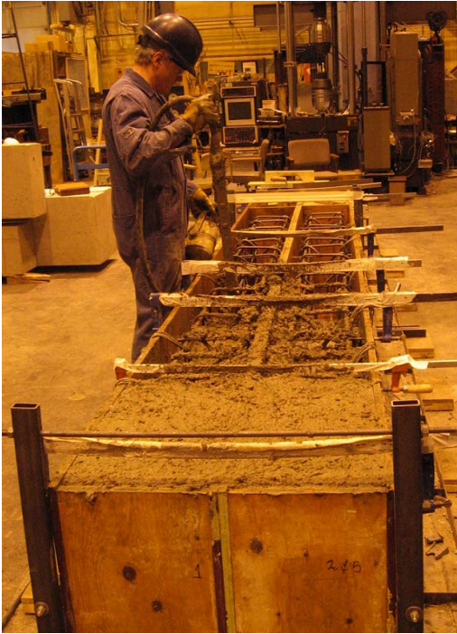
Figure 3-13 Vibration of the concrete during casting
