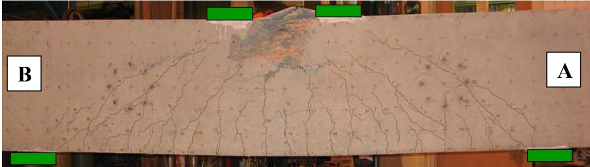
Figure 4-55 Specimen NS2-4 after failure
