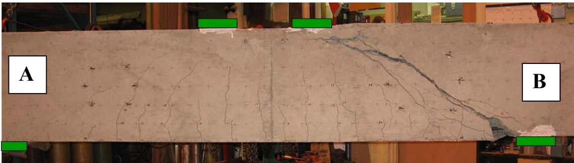
Figure 4-44 Specimen MW3-2 after failure
