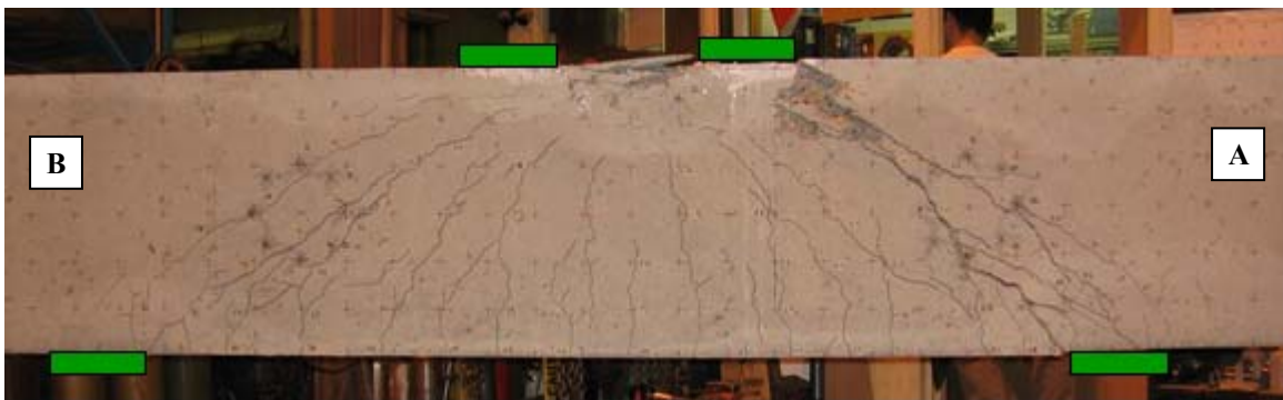
Figure 4-26 Specimen MS2-3 after failure
