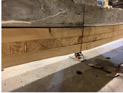
Figure 8.74: Rolling shear in specimen (#11) CLT4.5-C100-I5-45°-S250
