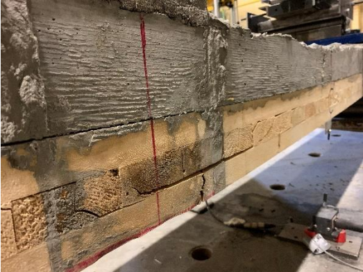
Figure 8.76: Rolling shear in specimen (#12) CLT4.5-C100-I0-30°-S250
