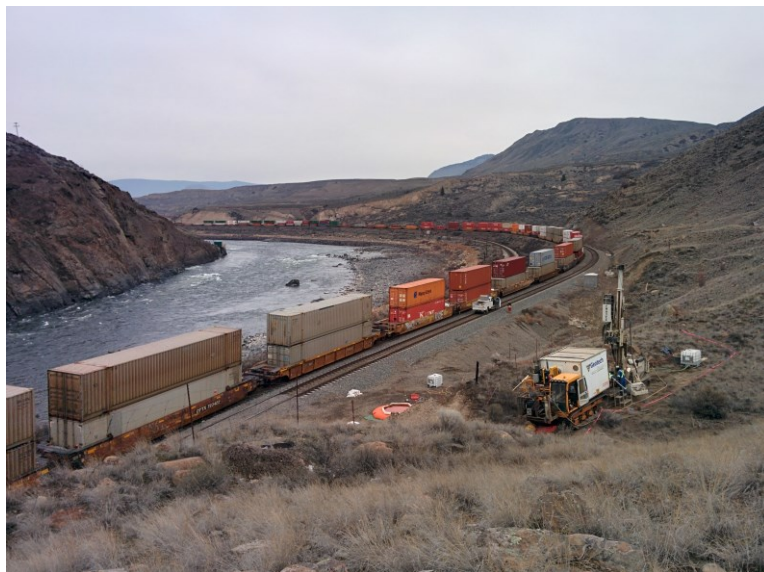
Figure 4.2. BH15-01 drilling location, looking north
