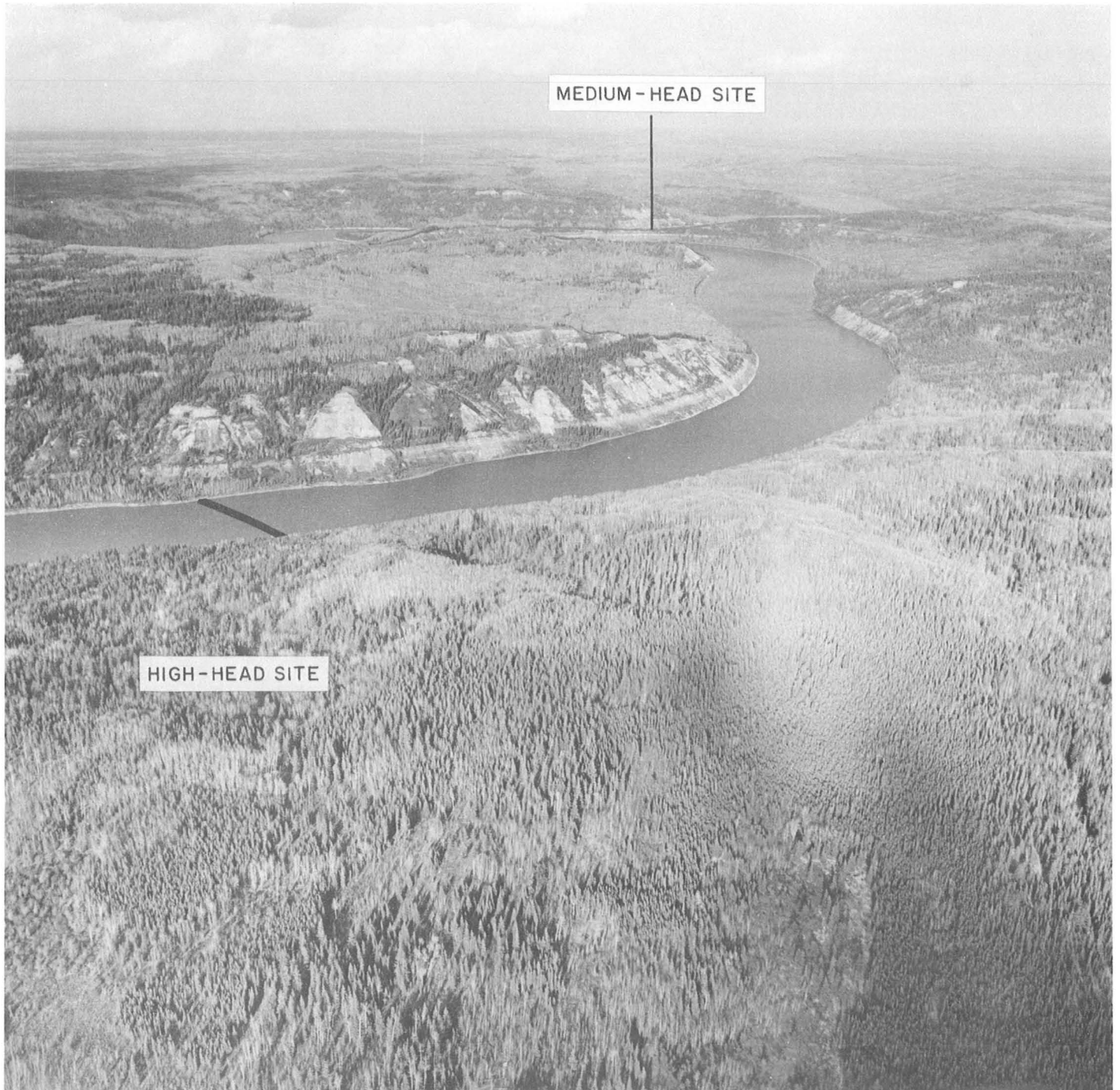
PHOTO 1. GENERAL VIEW OF DAMSITE STUDY AREA. THE ATHABASCA RIVER FLOWS TOWARDS RIGHT. NOTE ANCIENT MEANDER IN FRONT OF PRESENT CROOKED RAPIDS MEANDER LOOP.
