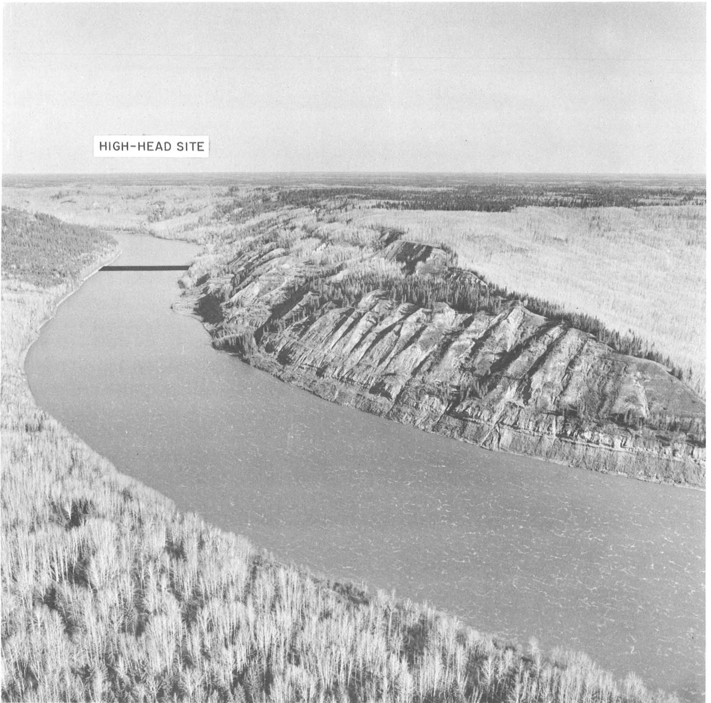
PHOTO 3. VIEW OF HIGH - HEAD SITE. THE ATHABASCA RIVER FLOWS TOWARDS RIGHT.
