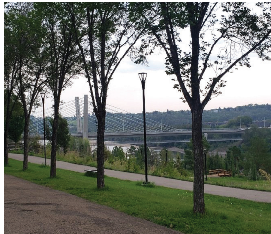
FIGURE 1a: Distance picture of the Tawatinâ Bridge [Quecke, E. August 15, 2023].
