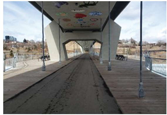
FIGURE 2a: View of Bridge Looking North from south end [Quecke, E. April 2, 2023]
