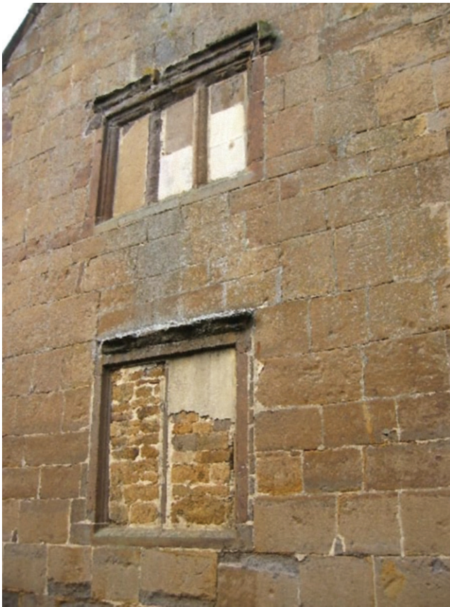
FIGURE 3: Example of a Defunct Window, Uppingham, UK. From "Window Tax Maybe?" by Kate Jewell, 2005, Geograph Project https://www.geograph.org.uk/photo/45159 . CC BY-SA 2.0
