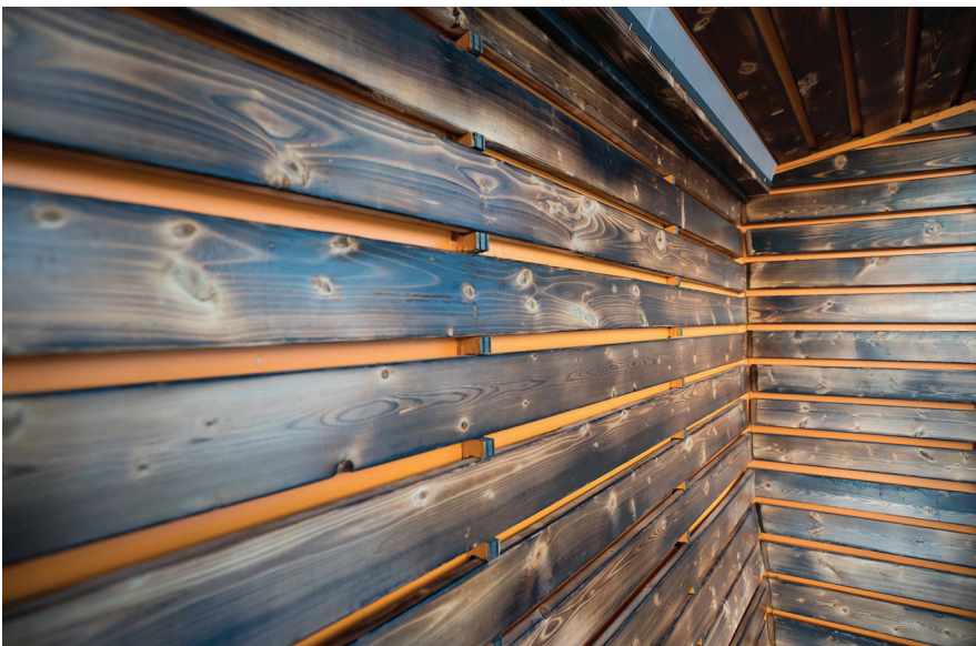
FIGURE 8: Interior of a warming hut made of charred pine and orange-painted plywood to reference a burning ember. Photo: Danielle Soneff. Photo provided by Danielle Soneff.
