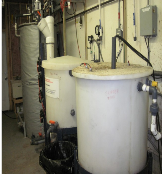
Figure A3. Mixing and Feeding Tanks
