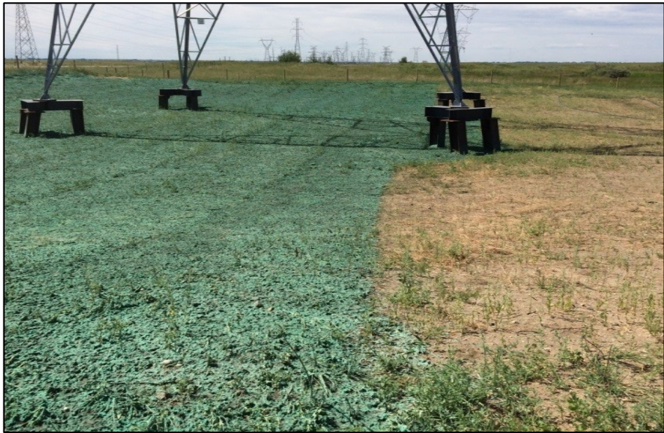
Figure 3-3. Sod-stripped tower site where soil was initially removed and replaced after tower construction (top), and vegetation was then re-established using a hydro-seeding treatment (bottom).
