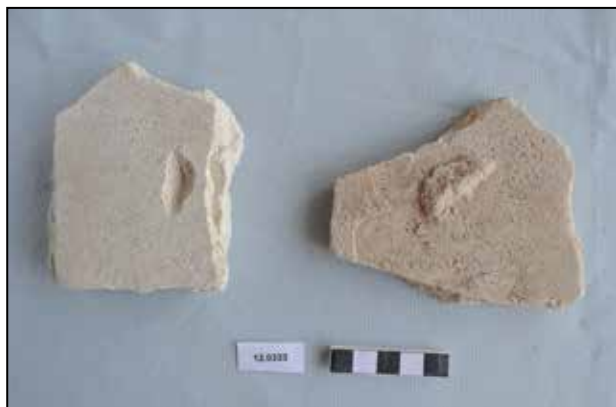
34. Top of an old layer of wall plaster punched (left) to key the underside of a new layer (right).
