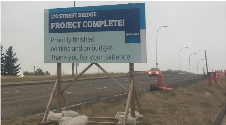
Figure 18: 170 Street over YHT - Bridge Rehabilitation
