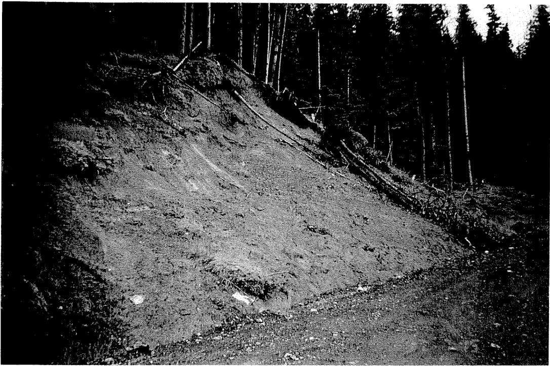
Figure 4 Earth slide in silty soils on the Hellroaring Road at 2.8 km (Figure 2)
