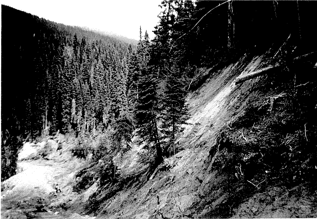
Figure 13 Morkill 45.7 km (Figure 2): Earth slide in sandy soils adjacent to road
