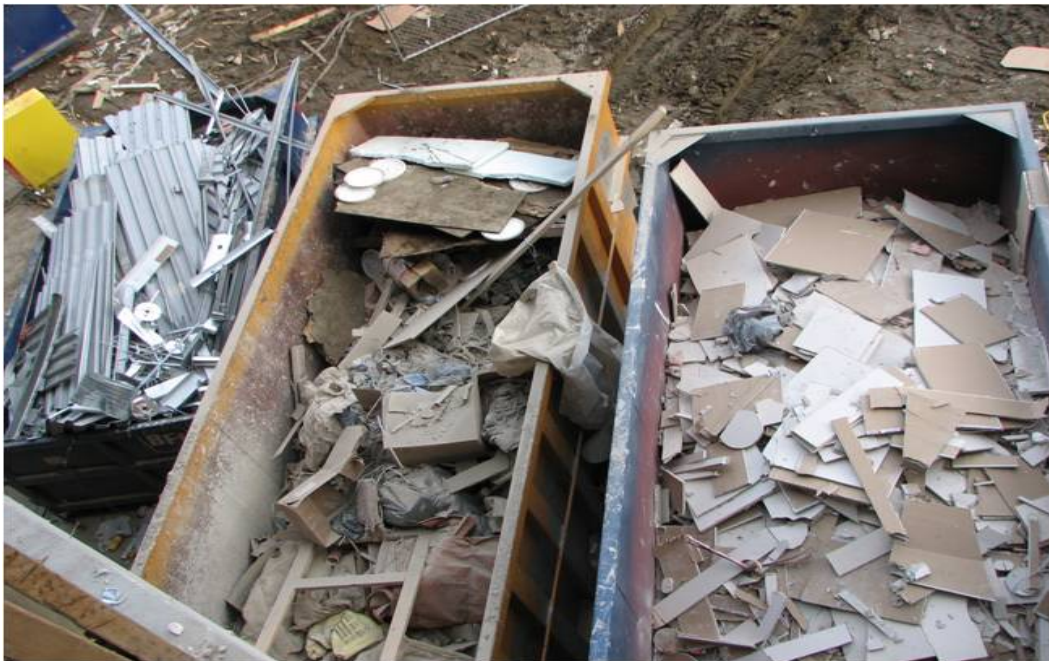
Figure 3. Drywall waste in residential constructions
