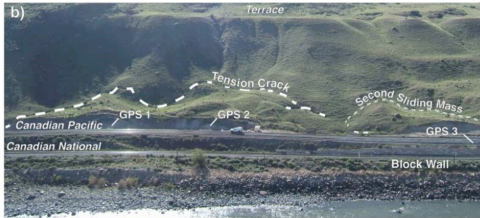
FIGURE 3-2. Ripley Slide Geometry including CN and CP railways and installed GPS on the site.
