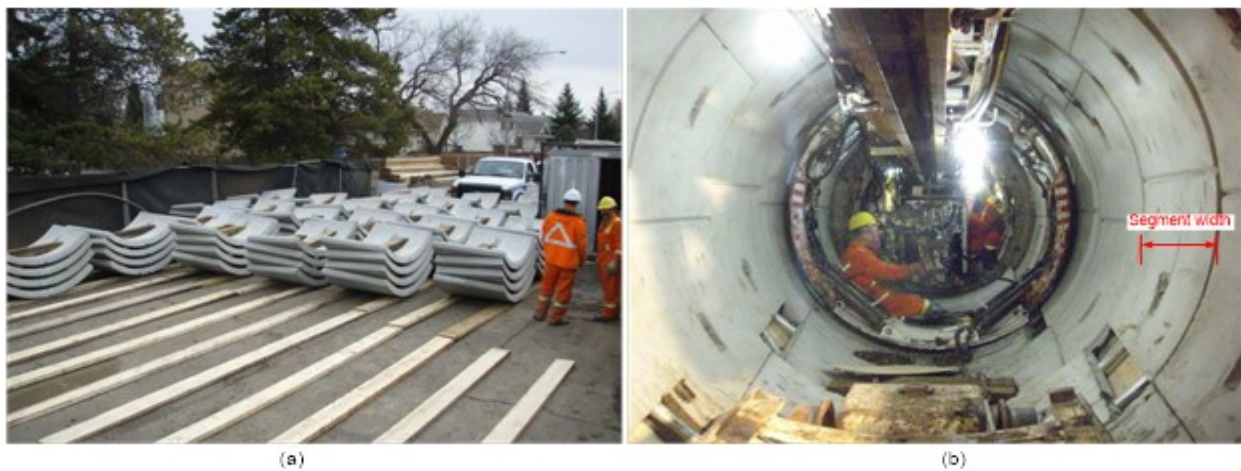
4 Figure 3.4: Segments for the WESS W13 Project: (a) Segments to the Site and (B) Segments in the Tunnel
