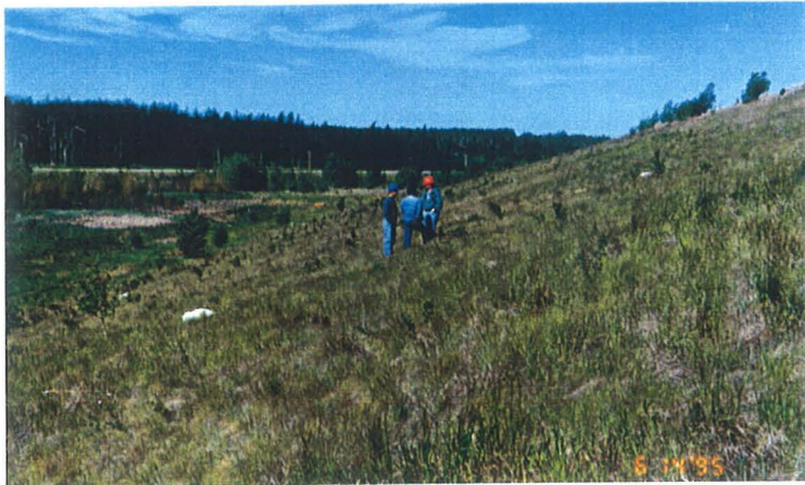
Grass cover providing effective erosion control on steep slope of reclaimed dyke.
