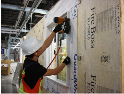
StationW9_2/W10_2:Window/door installation
