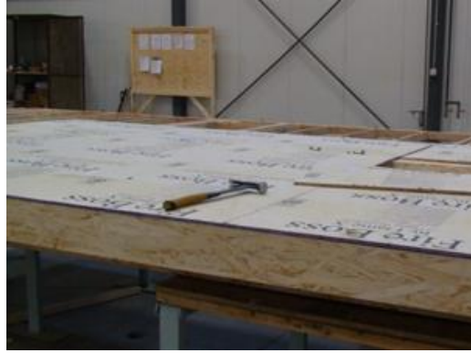
Station W4: Sheathing table
