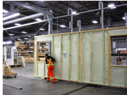
Station W9_1/W10_1: Buffer
