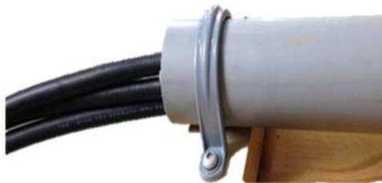
Figure 1.10: Inaccessibility of individual wires enclosed in conduit.
