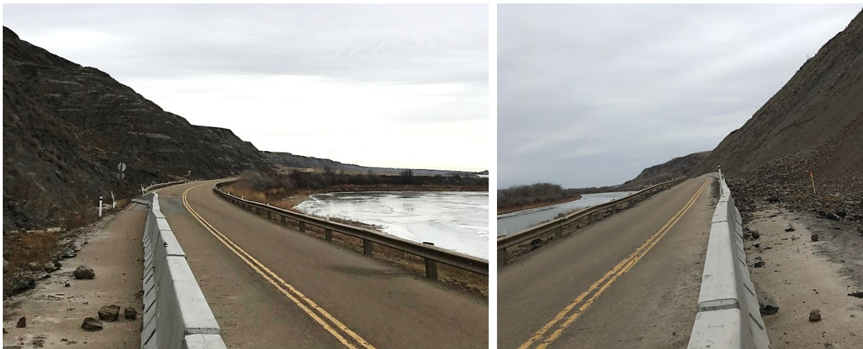
Figure 43: Jersey barriers partially closing one lane of Highway 837 at C018 site.
