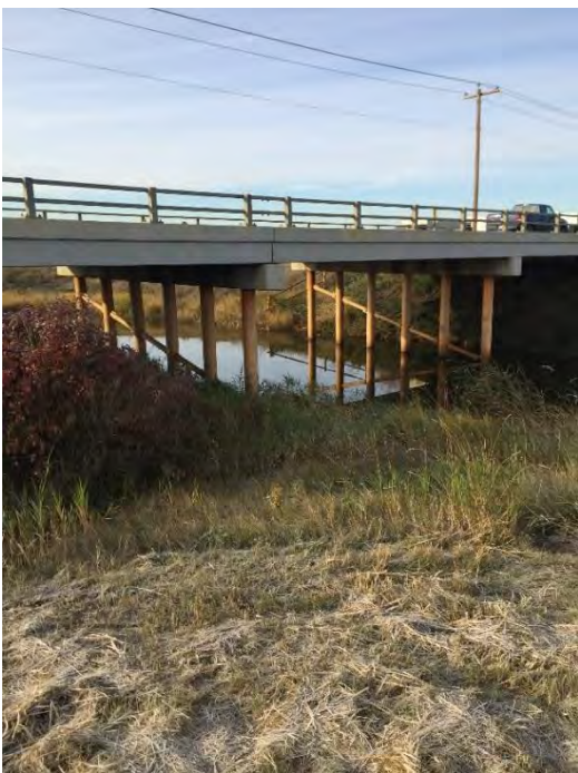
Photo 2-3. Blackmud Creek North of Township Road 510 (2016)
