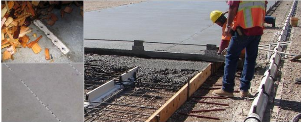
Figure 5.16: Air floor installation. Source: http://www.transformcompostsystems.com . Last accessed on September 15, 2011.
