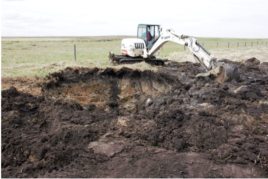
Figure 3 Construction of a ditch plug on the prairies.
