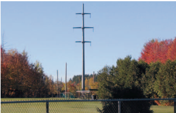
High-performance-concrete towers on the 120-kV Lafontaine–Paquin line (Laurentians).
