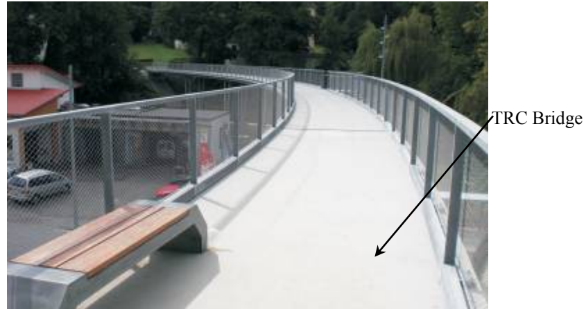
Figure 2.4- Pedestrian bridge made of textile reinforced concrete in Albstadt, Germany (Hegger et al., 2011)
