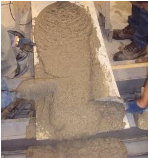
(a) Pouring and spreading of concrete
