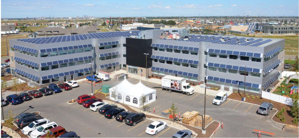
Figure 22: Solar PV system in Landmark Business Centre
