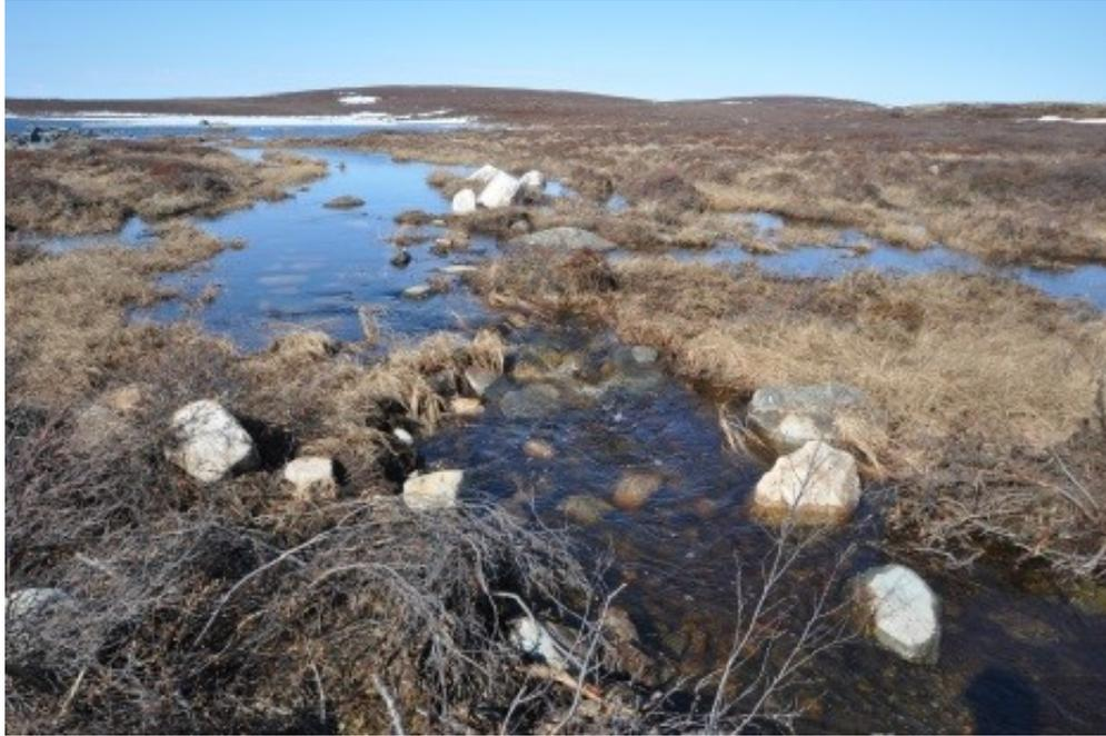
**Figure 3.8:** WIS Region A - Inlet - The upstream extent of construction is shown. A natural choke-point is located in the centre of the photograph. Upstream of the choke are several sub-channels which were blocked off with larger boulders to allow more flow into the main channel. This provides minimal hydraulic control during peak freshet as the reach functions as an active flood plain.
