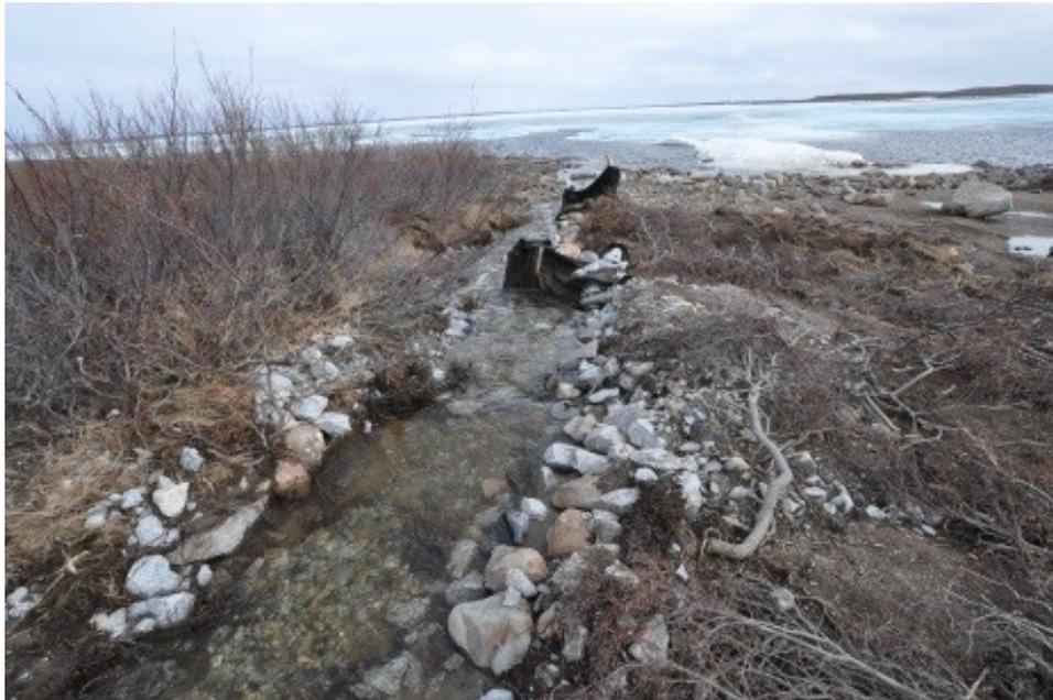
**Figure 3.14:** WIS Region G - Outlet - Looking downstream, Lac de Gras is shown in the background. This section was not modified from the natural channel as it was deemed suitable habitat and passable by fish. Silt fences are installed in the channel to reduce silt discharges into Lac de Gras from the disturbed sediment on the upper reaches of the newly excavated channel.
