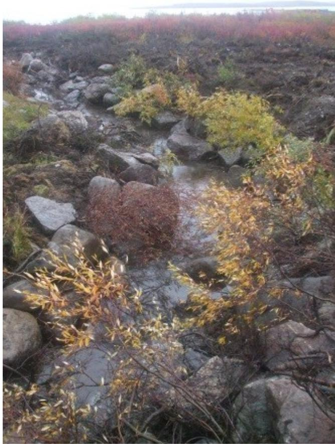
**Figure 3.10:** WIS Region C - Riffle One - Looking upstream, this section consists of a silt bed with a few larger boulders and willow vegetation on the banks to improve cover for fish habitat. During the first freshet period, additional silt was deposited in this reach due to the freshly excavated channel causing increased sediment transport.
