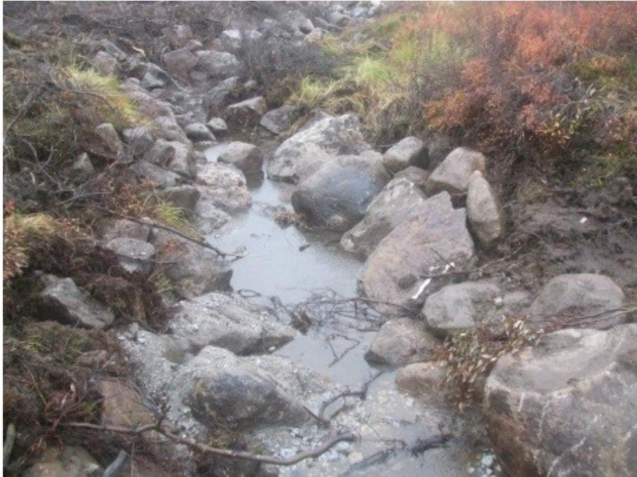
**Figure 3.11:** WIS Region D - Rock Ramp - Looking upstream, this section consists of a series of staggered boulders of various sizes with several choke structures in the foreground. Boulders optimize fish habitat suitability by creating additional flow variability, breaking up faster riffle flows with slower resting zones.
