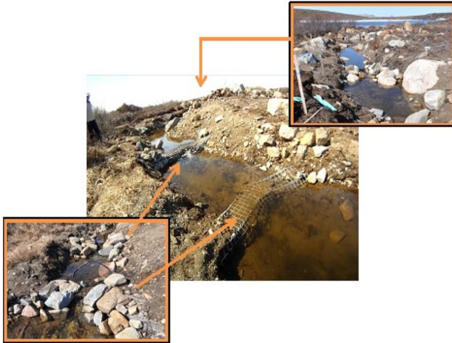
**Figure 2.5:** Image of M3S with original gabion structures at weirs four (left) and five (right); image is facing upstream towards M3L. Overlaid images depict the location and details of various retrofitted structures including weirs four and five (bottom left overlay) and weir two with additional minor boulder structures (top right overlay). Top right overlay image is located behind the bank in the main image and is not visible.
