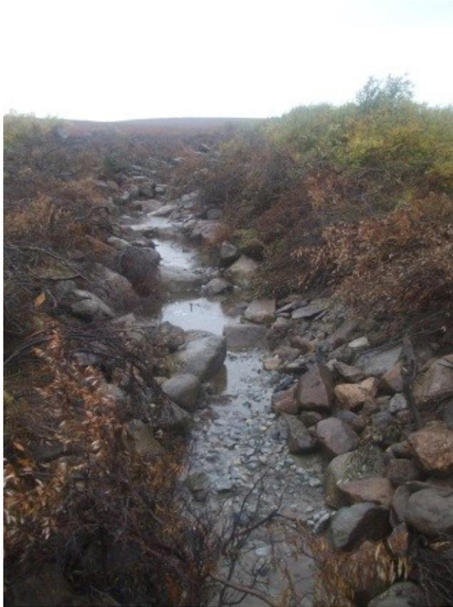
**Figure 3.9:** WIS Region B - Pool and Weir One - Looking upstream, the channel consists of boulders configured into weir and choke structures. The bed is lined with gravel and cobbles with willow vegetation on the banks to improve cover for fish habitat.
