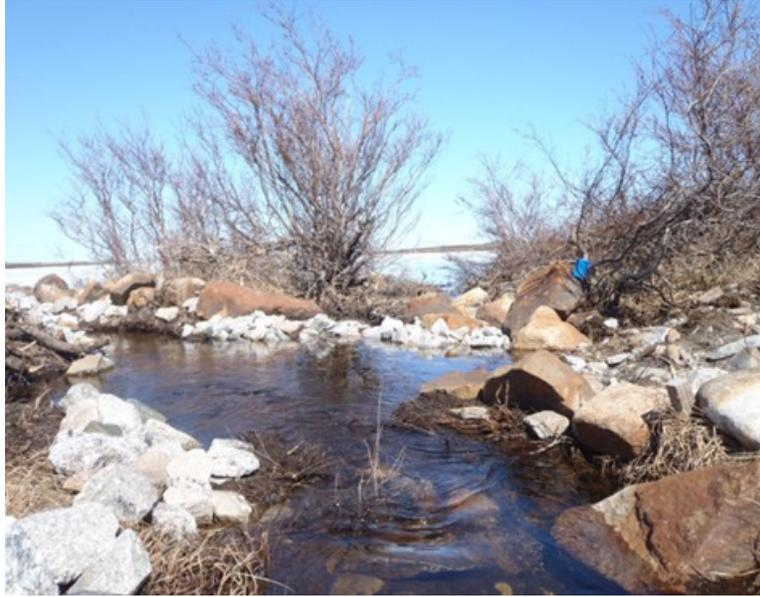
**Figure 2.6:** M2S choke-and-pool structure, facing downstream towards M1L. Preliminary evaluations indicated project goals were successful for this structure. A retrofit was not necessary unlike M1S and M3S. Fish were documented using M2S in 2012 and 2013.
