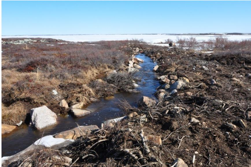
**Figure 3.12:** WIS Region E - Riffle Two - Looking downstream, this region is similar to Region C, consisting of a silt bed with a few large boulders. Substantial silt deposition occurred in this reach, altering the bed characteristics from the as-built channel. Photograph was taken several days after silt deposition declined. Channel characteristics changed over the first freshet period from variable and rocky to a more uniform and silted bed.
