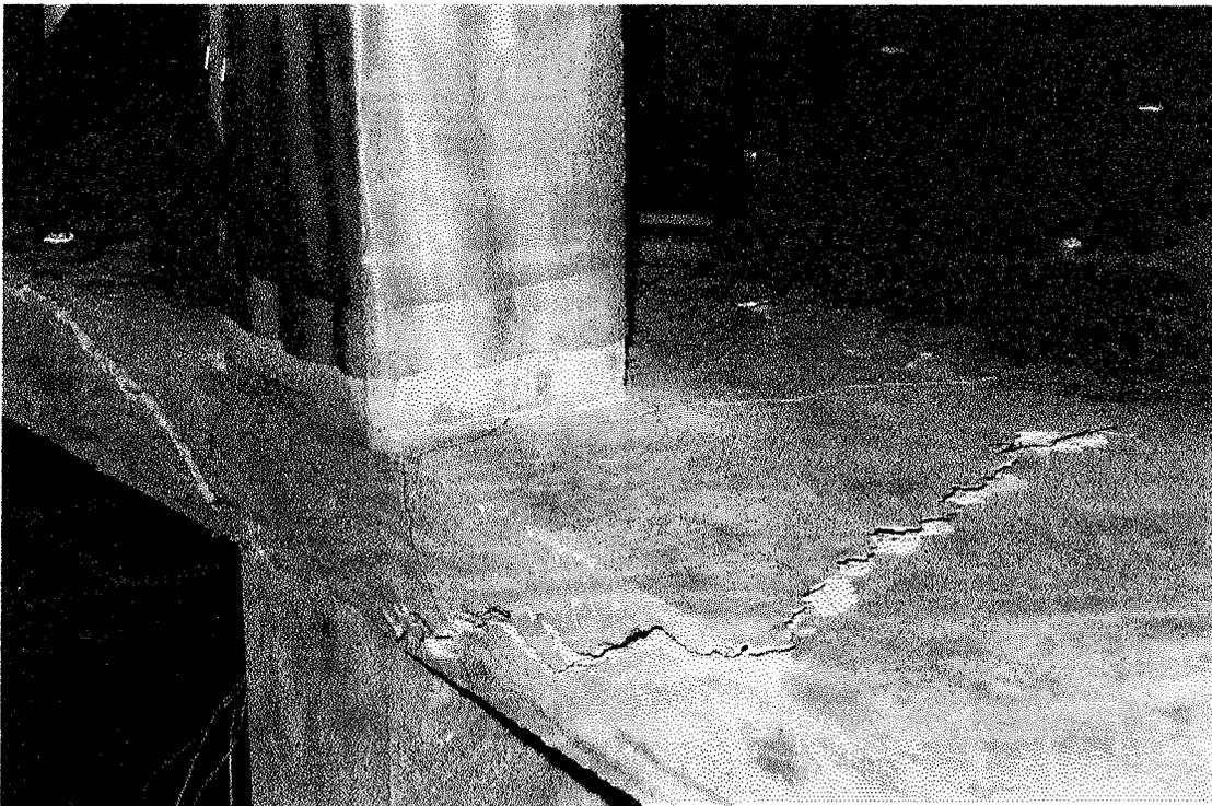
Figure 2.2 Typical punching failure of an edge connection
