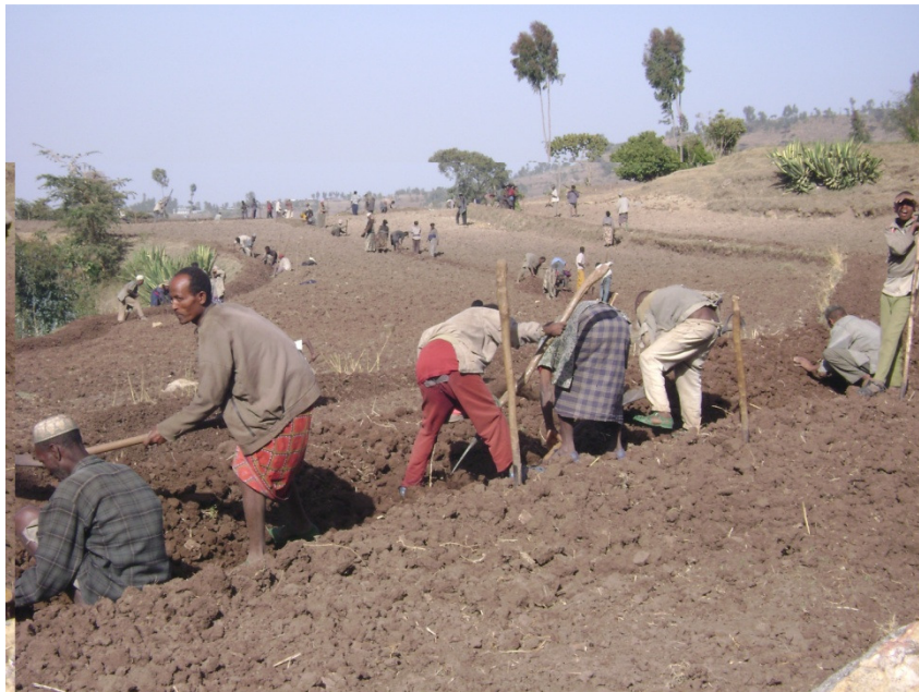
Plate 10: Building soil bunds in Misirāta on paid public labor mobilized from different villages
