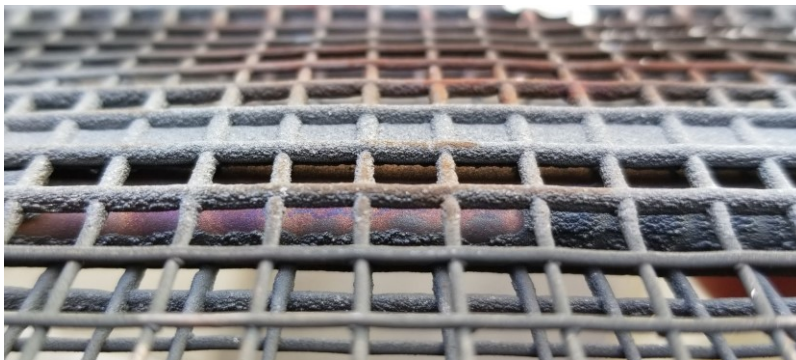
Figure 30: Coating delamination from tube surface, showing gap between mesh and tube
