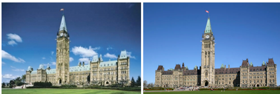
Figure 2.1: Canadian Parliament building. Left image: prior to restoration, right image: post restoration 4,5
