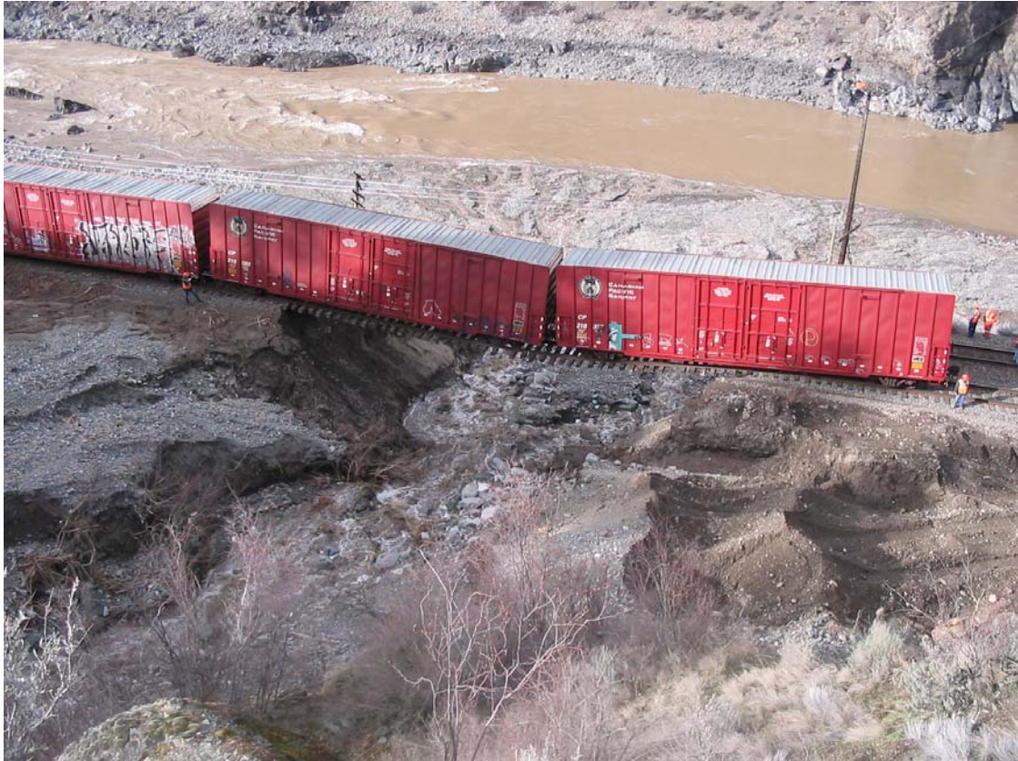
Photo 5.1 March 12, 2007, Lytton THOM 085.20 overland flow - gully erosion - debris flow event left the track skeleton over a 30 m length. A string of box-cars was stationary in the siding track at the time of the overland flow and is shown stranded over the unsupported track. The damage was caused by the bed-load and debris in the initial overland flow plugging the culvert. Subsequent gully erosion and debris flow erosion failed and eroded the track embankment spanning the gully.
