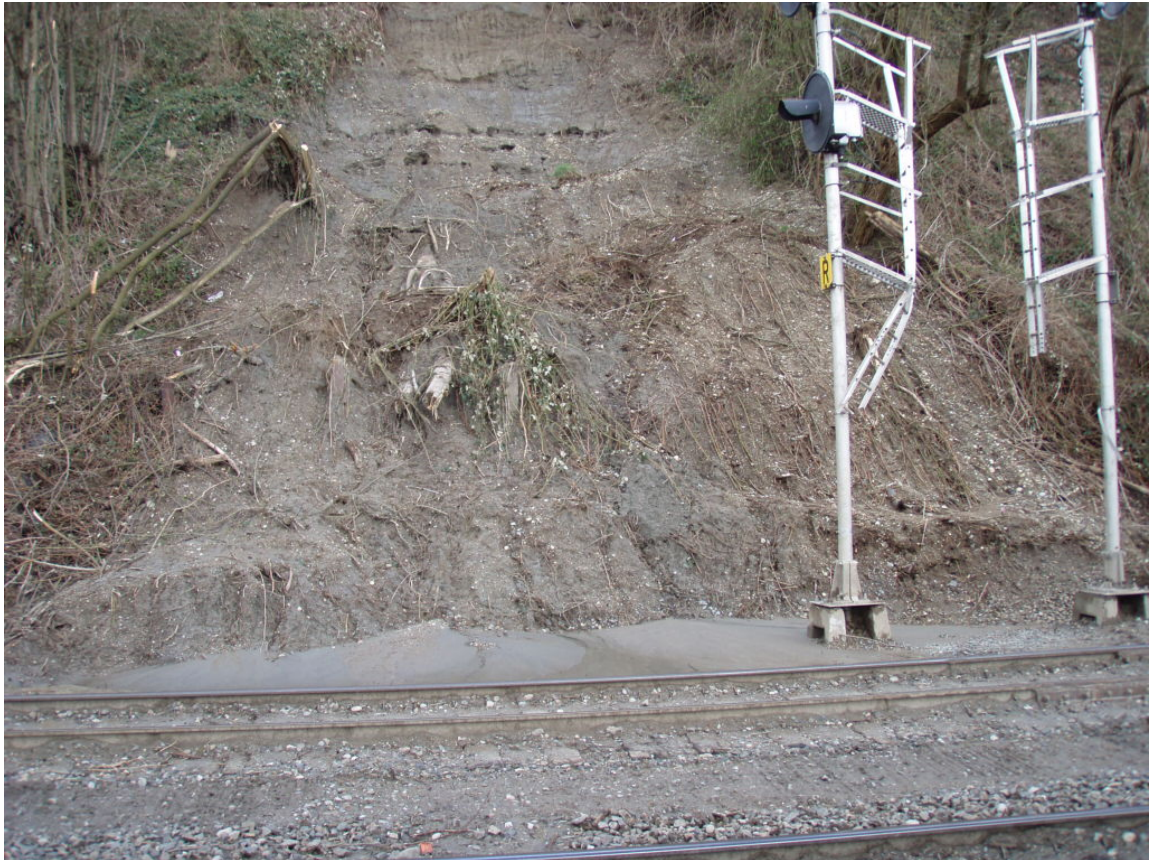
Photo 4.3 Photo is of CASC 103.41 following the March 24, 2007 earth slide at this location. The debris has been removed from the track. The flow from the interbedded silty clay and fine sand layers is illustrated by piping points at, below, and above the elevation of the black signal-light housing. The miniature alluvial fans of non-cohesive sand in the ditch to the left of the signal post are evidence of piping of the sand seams. Photo by Alastair Grogan
