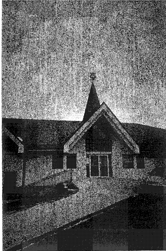
Figure 4.2: Photograph of First Mennonite Church
