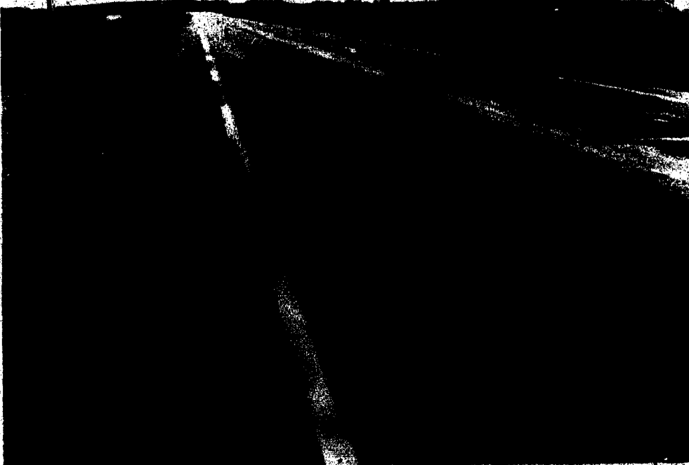
Photo E-8 Highway 45:06B. Example of overlaid full-depth pavement. Pavement age - 17 years. Overlay age - 10 years. Medium traffic.
