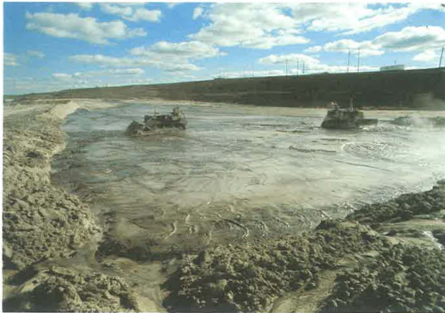
Figure 1.3.3-17 Dozers constructing tailings dyke cells.
