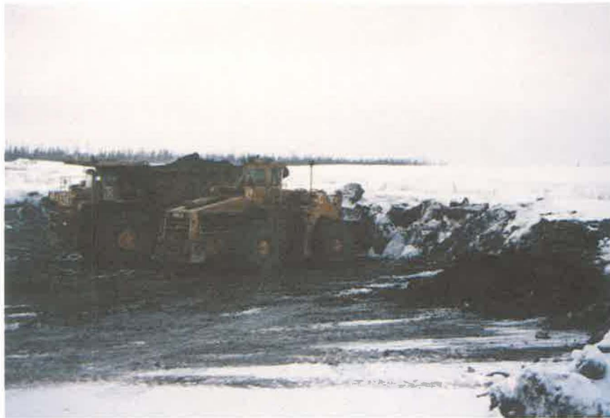
Figure 1.3.3-3 Excavating muskeg during the winter with front-end loader and hauling with off-highway truck.
