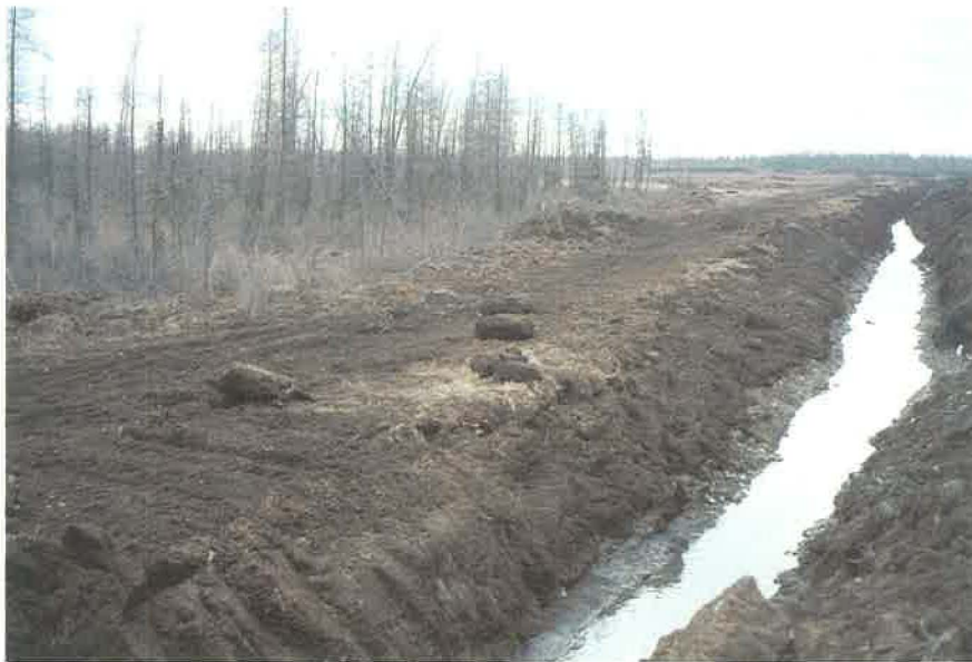
Figure 1.3.3-1 Dewatering ditch in muskeg.
