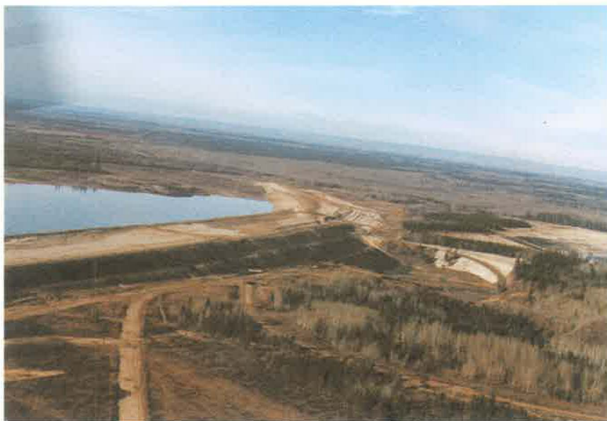
Figure 1.3.3-23 The earth-filled starter dam of an out-of-pit tailings pond.
