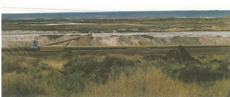
Figure 1.3.3-22 Tailings pipelines alongside a cell being constructed at the base of the tailings pond dyke.
