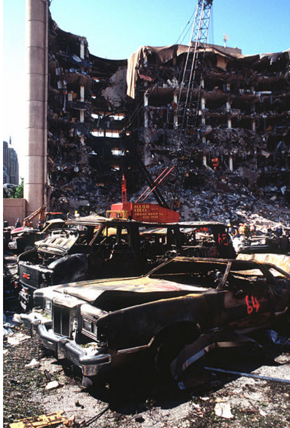
Figure 1.7: Alfred P. Murrah Federal Building, Oklahoma City, USA (NIST 2005)
