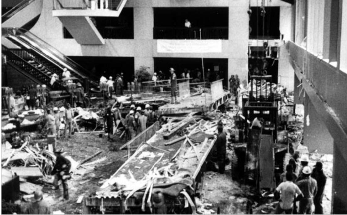
Figure 1.5: Hyatt Regency Hotel Skywalks, Kansas City, USA
