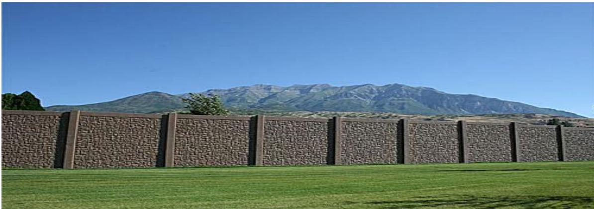
**Figure 17: Prefabricated Sound Barrier Wall (AFTEC, 2010)**
