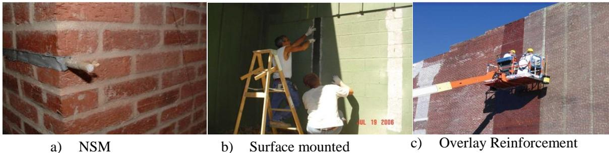
**Figure (2): Different technique of installation of FRP**
