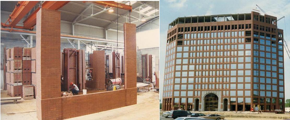
**Figure 3: Prefabricated Panels and Full Scale Illustration of the Columbia Center Tower (Building the Future, 2003)**
