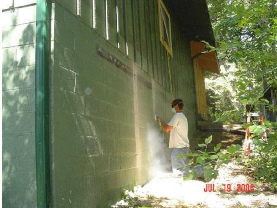
**Figure (15): Surface preparation of the wall**
