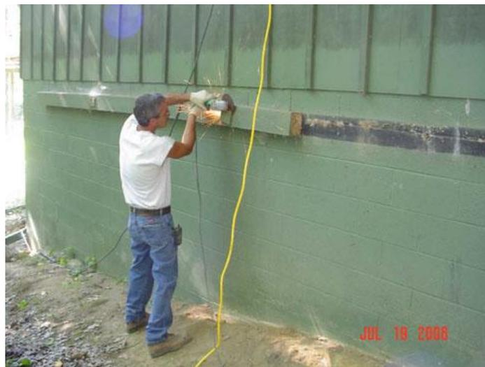
**Figure (10): Removal of the wood waller**
