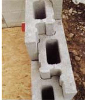
**Figure 12 - Sparlock Interlocking Block wall (Sparlock Technologies, 2010)**
