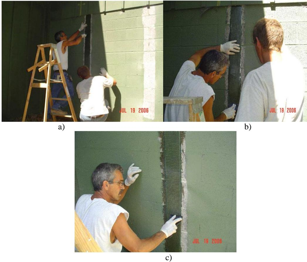
**Figure 17: Mounting the CFRP strip to the wall.**
