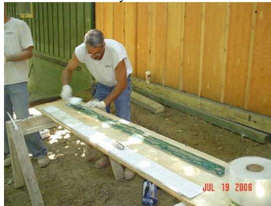
**Figure (16): Application of the epoxy paint to the CFRP lamination**
