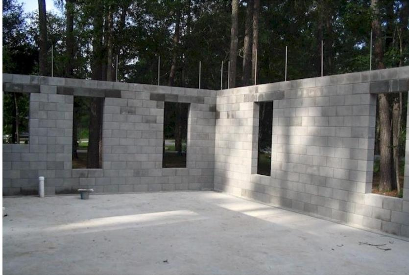
**Figure 6 - Completed building envelope for FlexLock house in Magnolia, TX (Cercorp Initiatives, 2010)**
