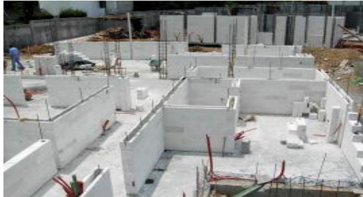
**Fig. 5.11 AAC Block Construction on Concrete Footing Base** <sup>(3.1)</sup>
