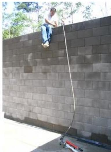
**Figure 7 - Post-tensioning of wall anchors for FlexLock house in Magnolia, TX (Cercorp Initiatives, 2010).**
