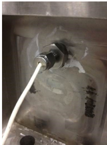
Figure 3-24 Closure of the tapping after installation of Kulite pore pressure transducer.
