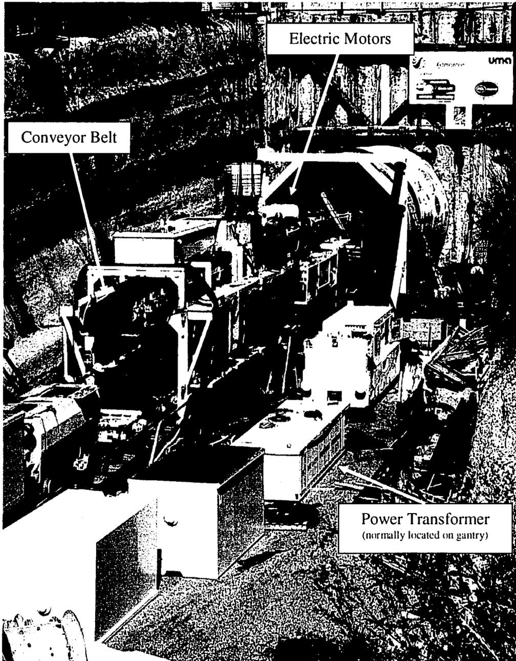
Figure 2-12 Partially Assembled Gantry, August 12, 2003
