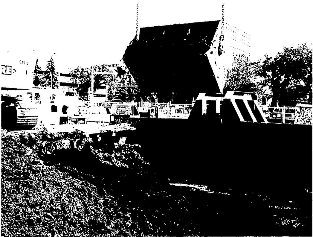
Figure 4-1 TBM spoil being dumped into muck bin.
