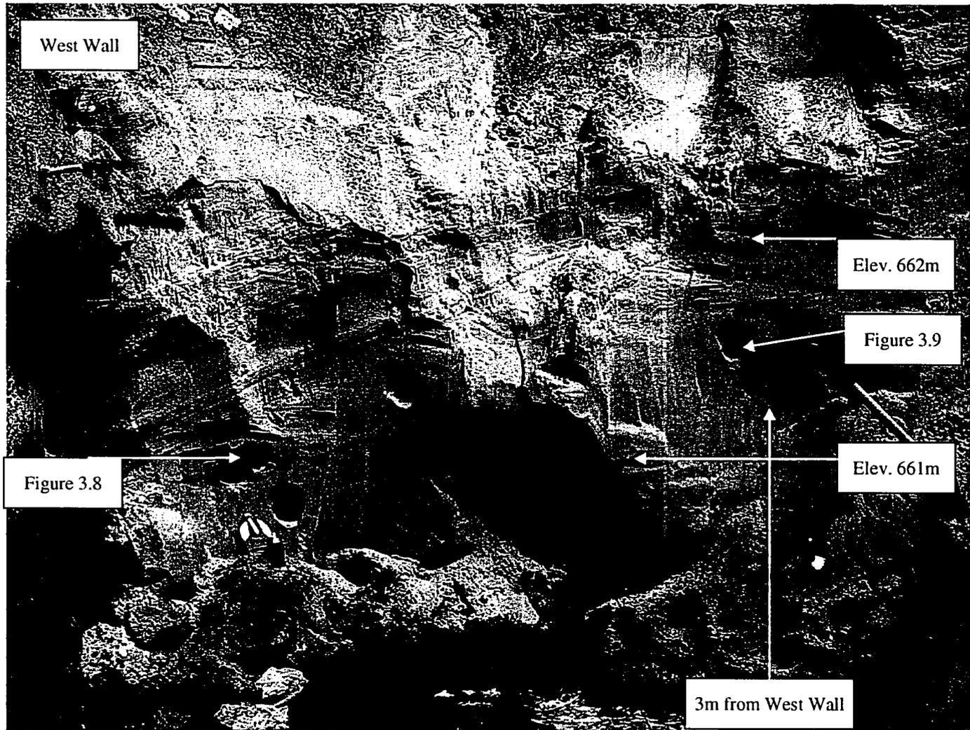
Figure 3-6 Mapping of exposed face of Outwash Sands and Silts during portal excavation, south facing along West Wall
