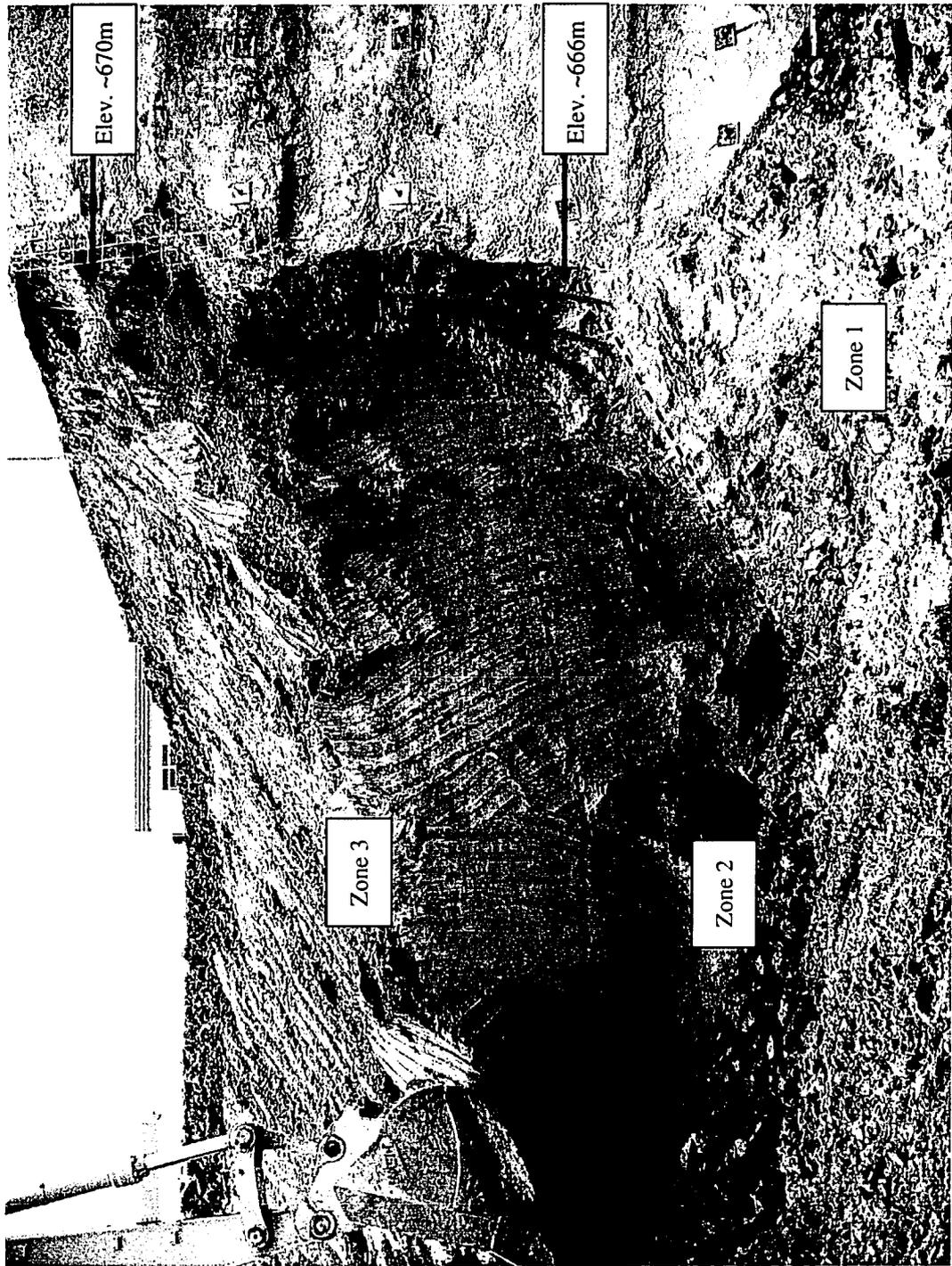
Figure 3-4 Transition zone between Outwash Sands and Silts and Lake Edmonton Clay.
