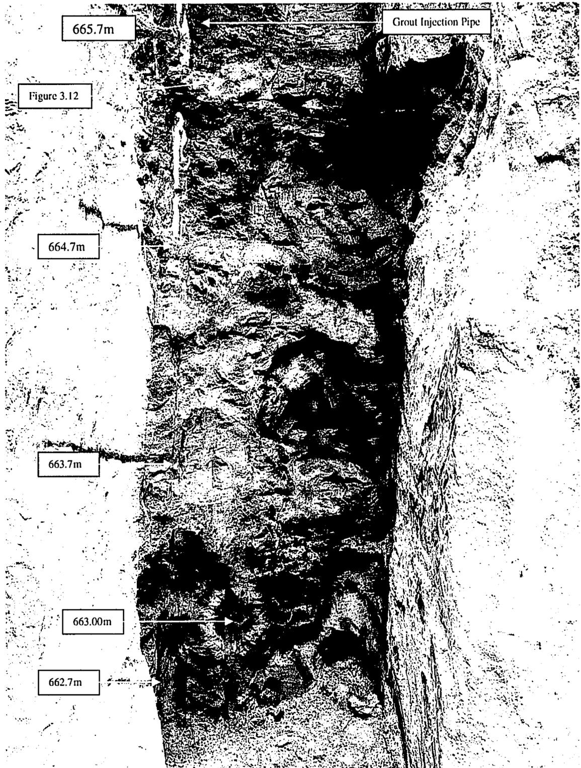
Figure 3-12 Exposed face of chemically grouted soil.
