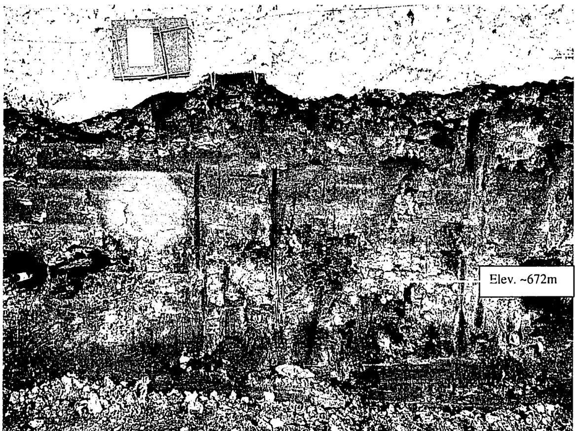
Figure 3-3 Exposed face of Lake Edmonton Clay during portal excavation, soil anchors present in left of photo at Elev. 672m.
