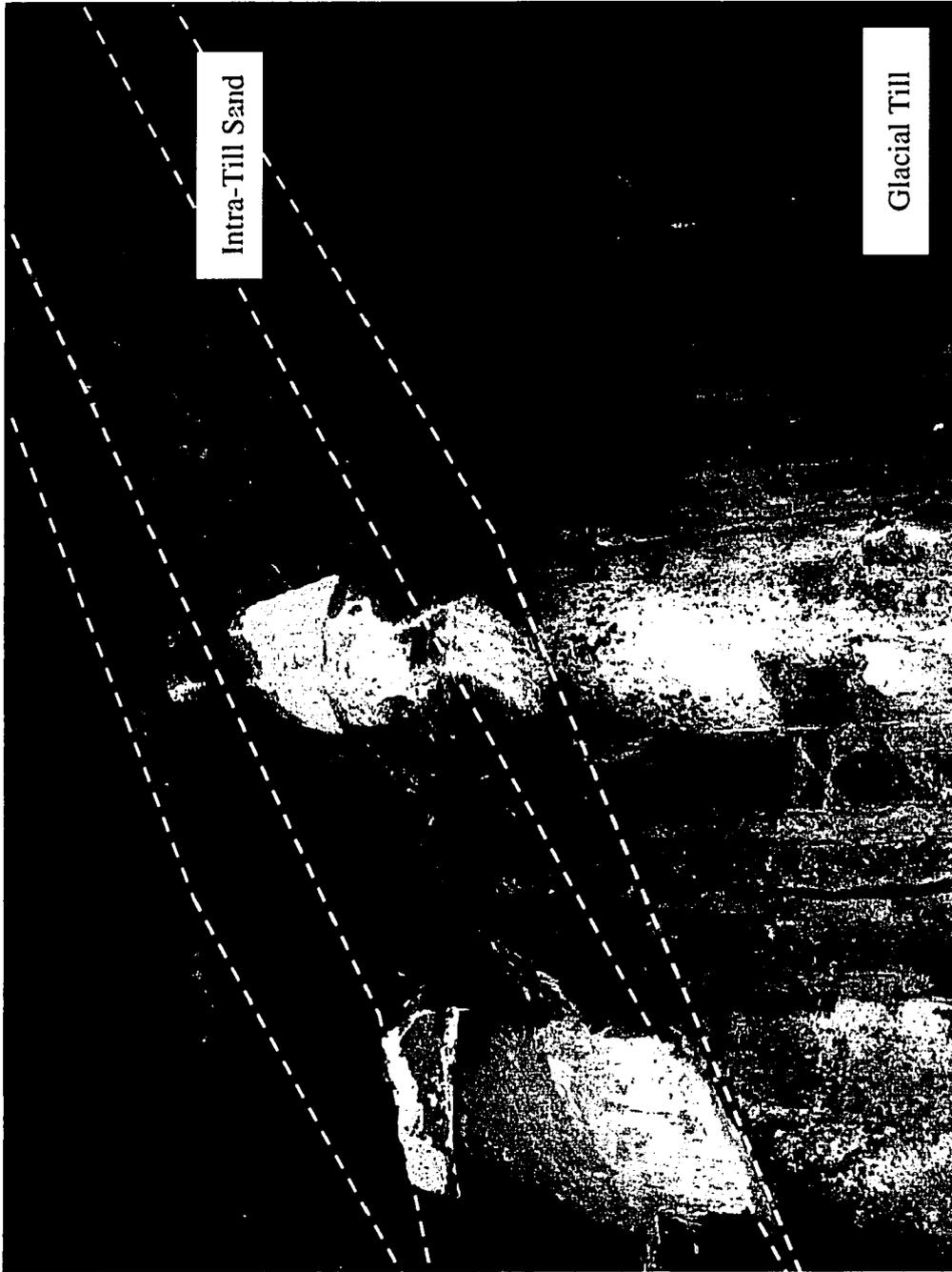
Figure 3-23 Intra-Till Sands striking across tangent pile wall in removal shaft (elev. ~657)
