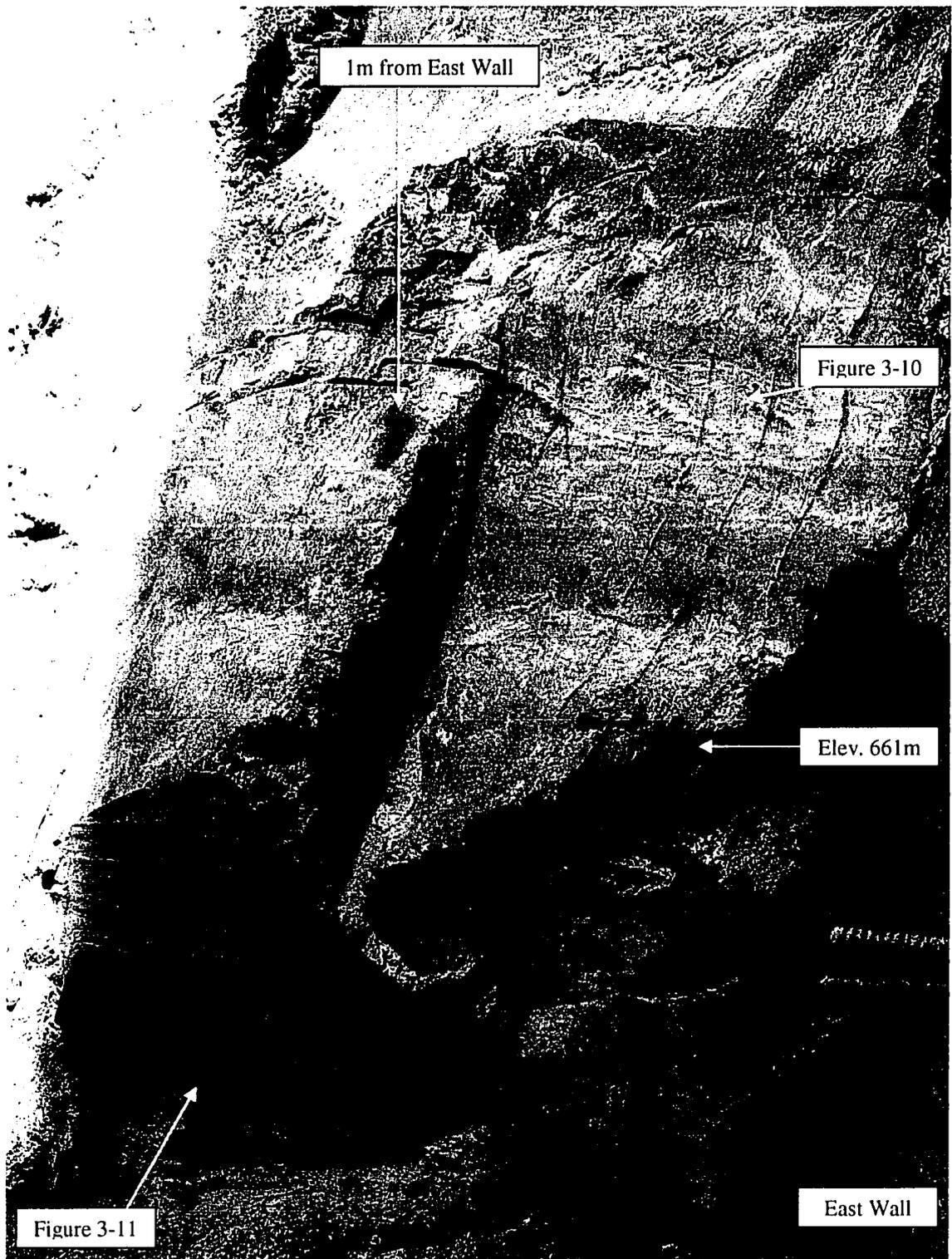
Figure 3-7 Mapping of exposed face of Outwash Sands and Silts during portal excavation, south facing along East Wall.
