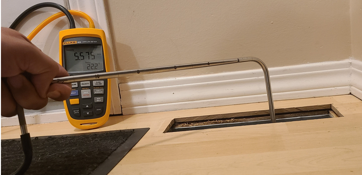
Figure 3.3: Measuring air velocity for each supply air register.
